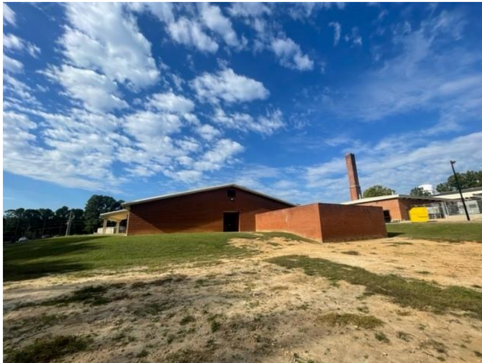
Figure 2: View from B-05, Center of proposed building addition
