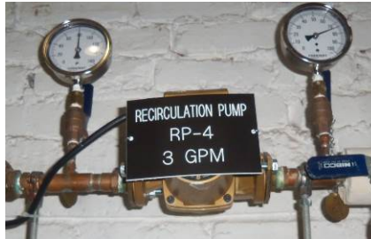
DHW-1 and recirculation pump
