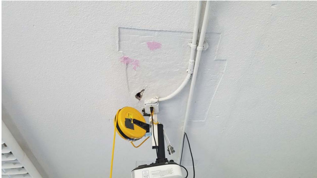
Example of Asbestos-Containing Ceiling Texture
