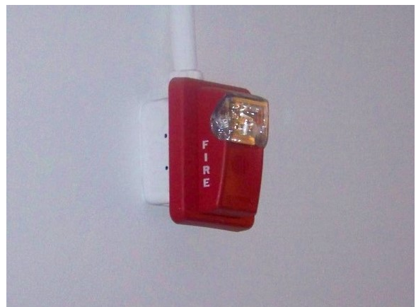
Horn/strobe for alarm notification
