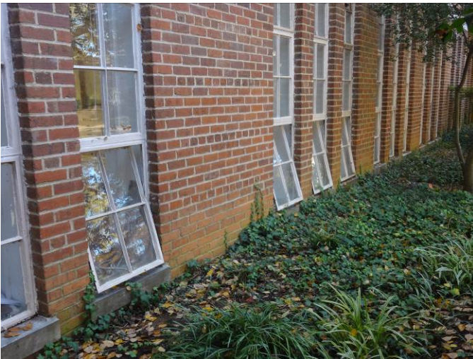
Typical single-glaze steel-framed window (L) and insulating panel at second floor (R)
