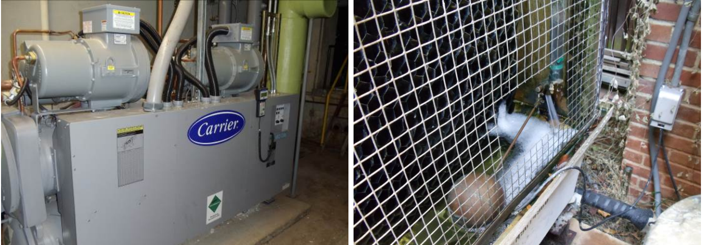
Carrier chiller to left, float switch and water feed for cooling tower to right.
