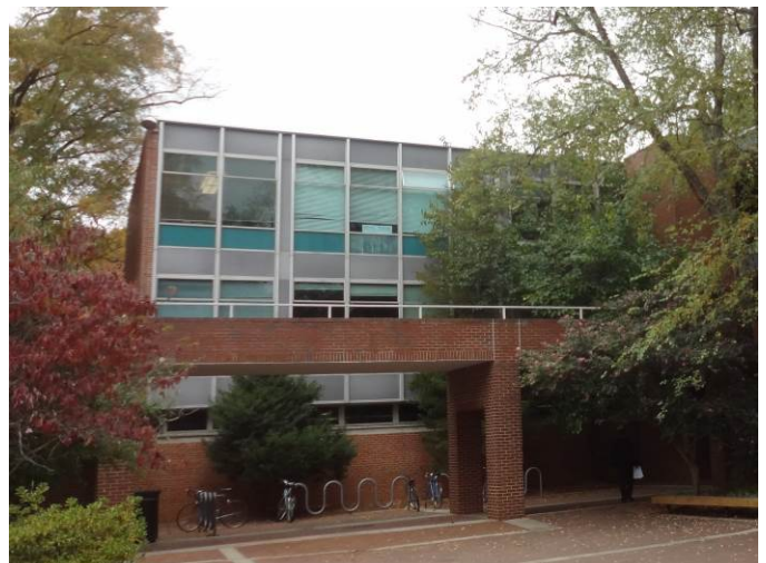
Clear and spandrel glazing at the north addition is single-pane throughout
