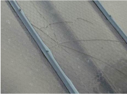
Broken wire-glass at rooftop, broken glass and dirt at ceiling plane of skylight and at oculus
