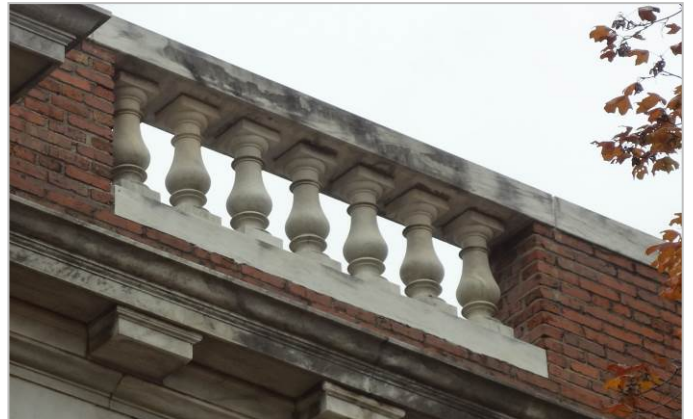
Marble accents and cornice at parapet; note stains and mortar loss
