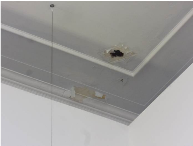
Water damage at plaster ceiling and molding in Design Library
