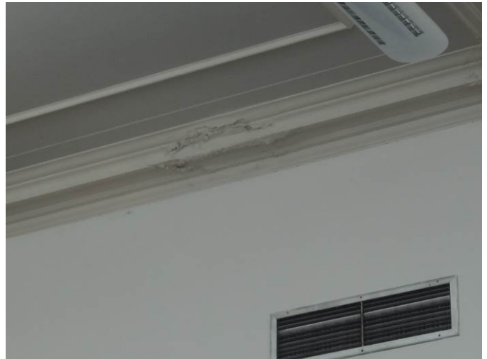
Water damage at plaster ceiling and molding in Design Library
