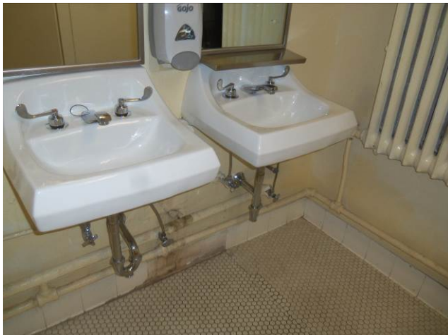
Antiquated hand wash sinks/fixtures and uninsulated piping under
