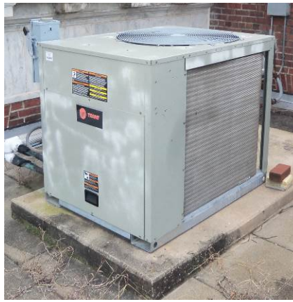
Condensing unit for AHU-2, above; AHU-2 right.
