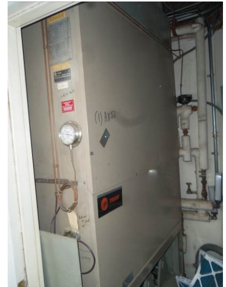
Condensing unit for AHU-2, above; AHU-2 right.
