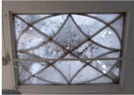
Broken wire-glass at rooftop, broken glass and dirt at ceiling plane of skylight and at oculus
