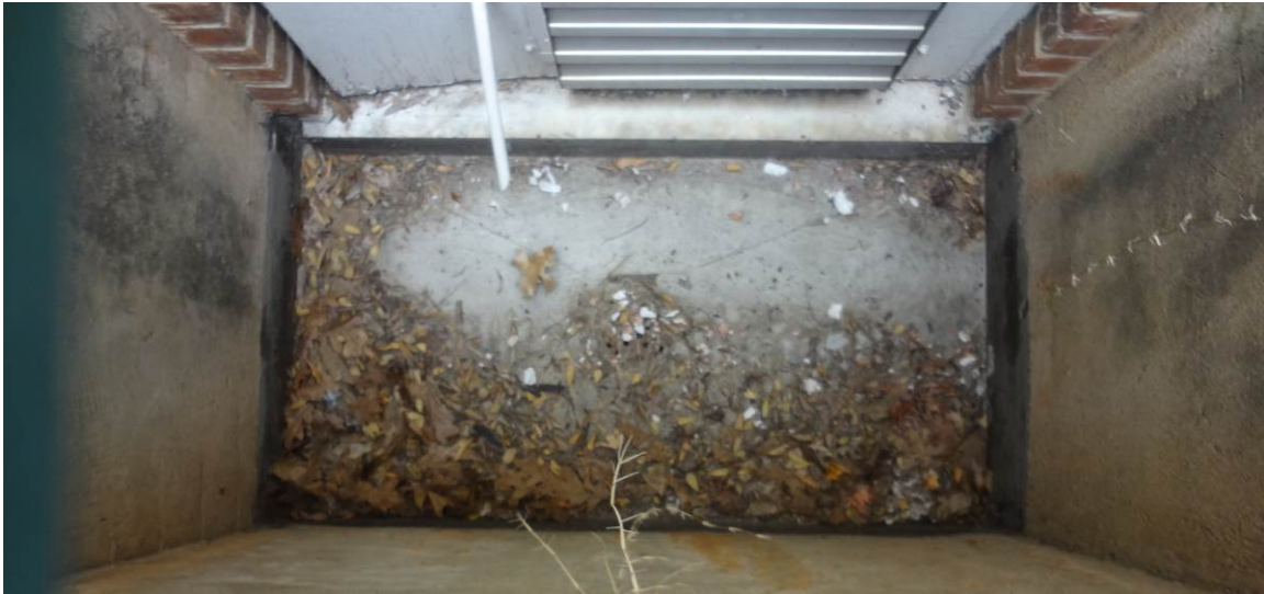
Leaves and debris in window well
