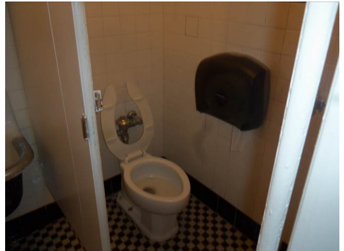
Non ADA compliant stall and non-low flow toilet fixture
