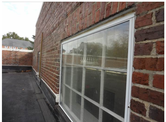
Typical single-glaze steel-framed window (L) and insulating panel at second floor (R)
