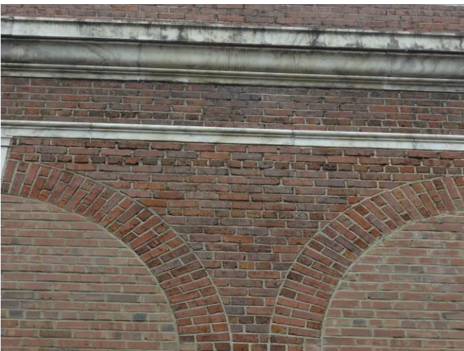
The arched upper portions of the west-facing reading room's windows were removed and infilled with brick
