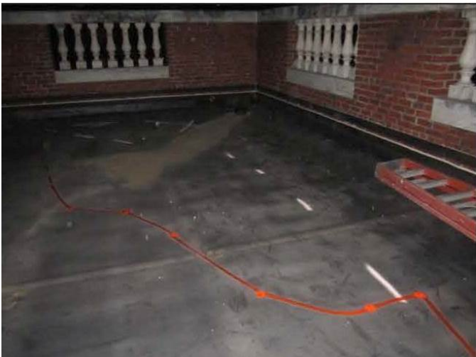
Stretched membrane at center block, painted line indicates extent of water infiltration and damaged insulation beneath membrane (L) confirmed by infrared testing (R)
