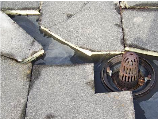
Broken LG boards at north wing (L), ponding at south wing (R)
