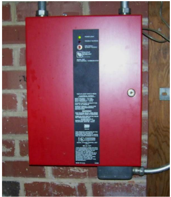
Silent Knight digital alarm communicator
