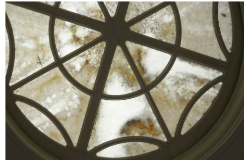
Broken wire-glass at rooftop, broken glass and dirt at ceiling plane of skylight and at oculus
