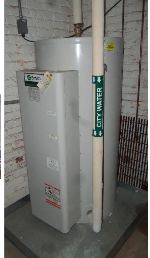
DHW-1 and recirculation pump
