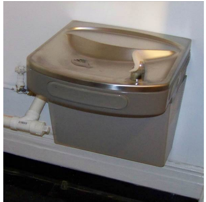
Examples of ADA non-compliance: hand rails that do not transition smoothly from one level to the next, and an obsolete design single-height drinking fountain.
