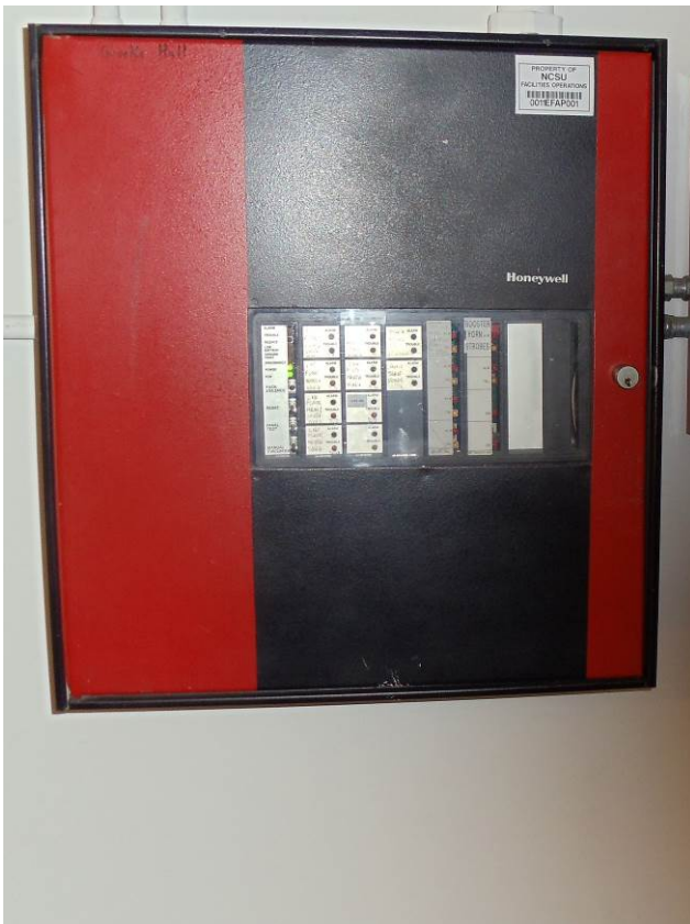
Honeywell FS90 fire alarm control panel
