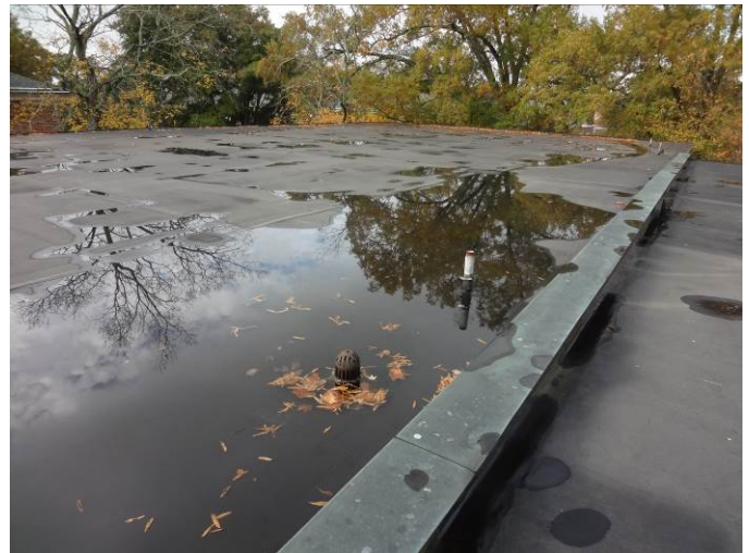
Broken LG boards at north wing (L), ponding at south wing (R)
