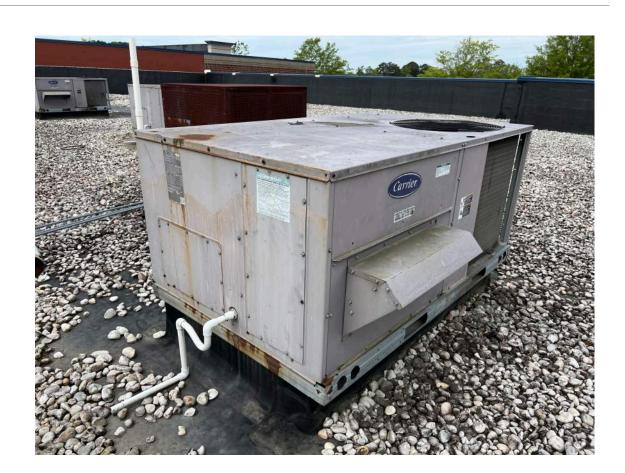
RTU-8 Capacity - 4 Type - HP
