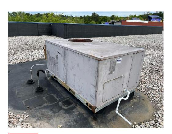
RTU-9 Capacity - 5 Type - HP
