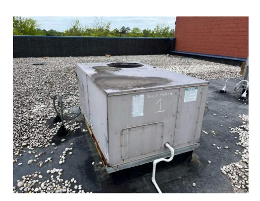
RTU-2 Capacity - 4 Type - HP
