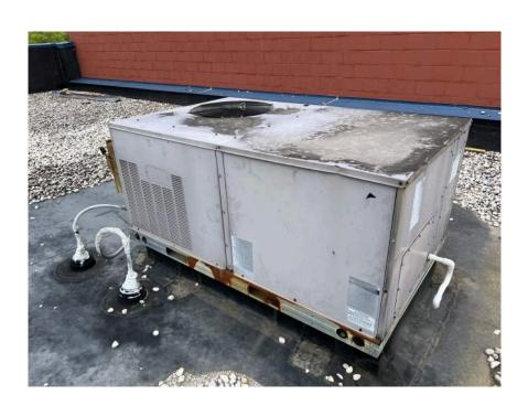
RTU-1 Capacity - 4 Type - HP
