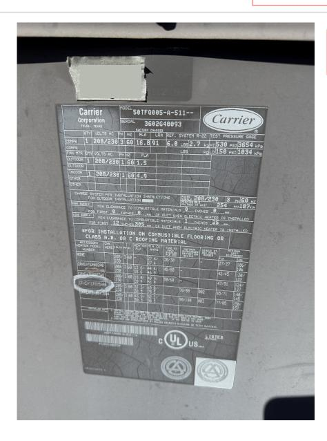
RTU-23 Capacity - 4 Type - HP
