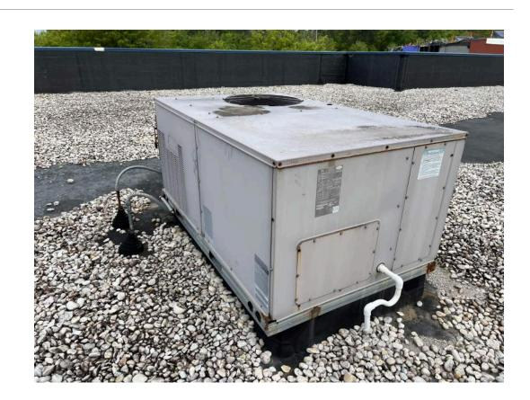
RTU-10 Capacity - 4 Type - HP
