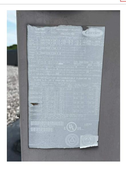
RTU-5 Capacity - 7.5 Type - HP
